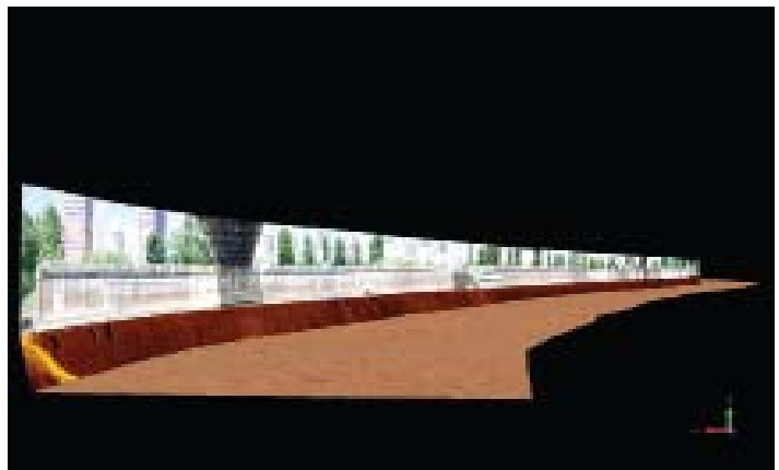
More sonar views of the harbor seawall along the Willamette River.
